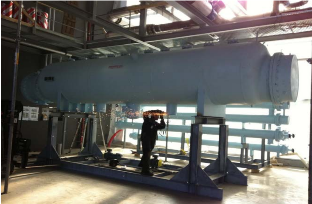
Figur 36: NH 3 spray fordamer for 5 MW varmepumpe, [Vedlegg 2].
